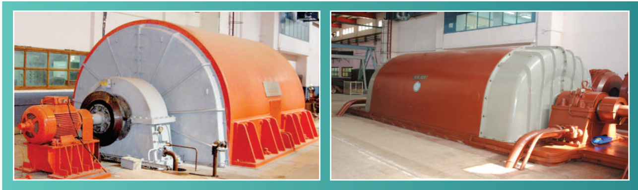
Two Nos., 1500MVA, 12.5 kV, 69 kA, 3 Phase SHORT CIRCUIT GENERATOR
