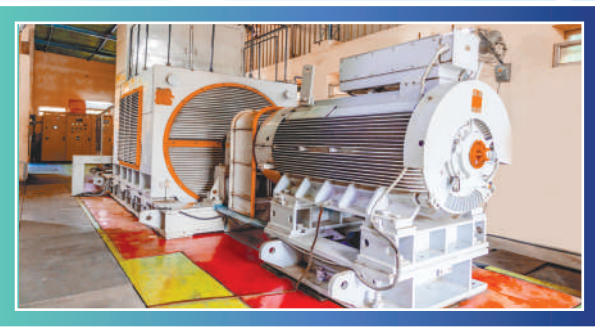
50MVA, 12kV Short Circuit Generator
