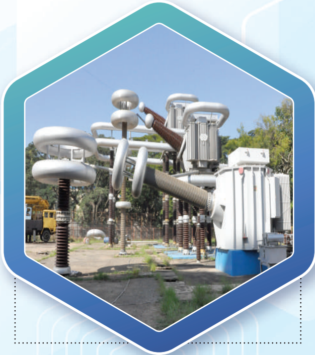
1800 kV, 2000 kVA cascade transformer
