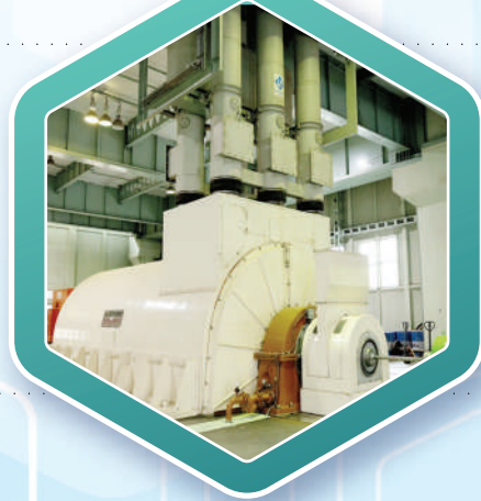
2500MVA Short circuit generator
