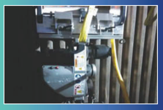
Robotic System for Boiler Water Wall Tube Inspection
